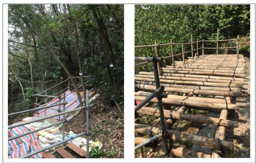
Reference photos - For protection of the vegetated slopes, temporary bamboo and metal working platforms for the drill holes will be formed with least disturbance to the surrounding environment.
