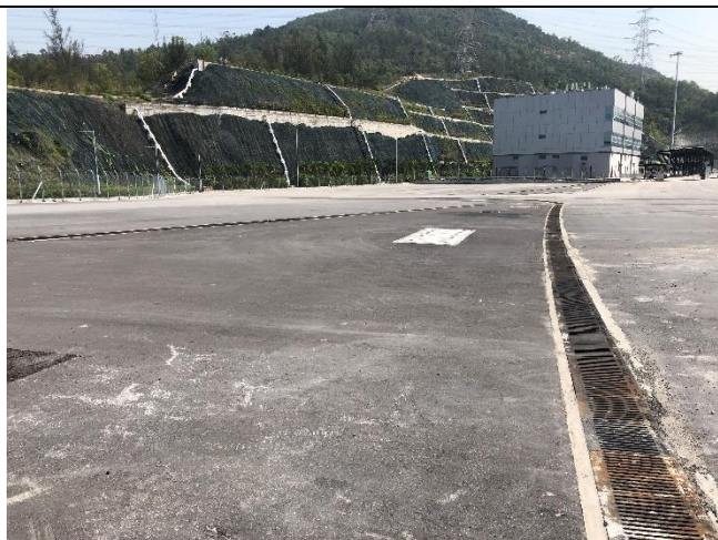
Photo 7: Drainage within the Site A
