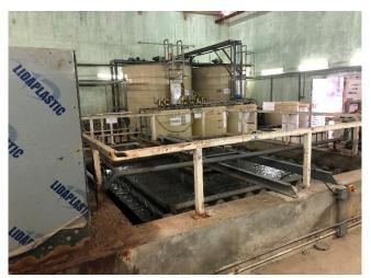
Photo 35: Reaction Tanks within the Wastewater Treatment Plant
