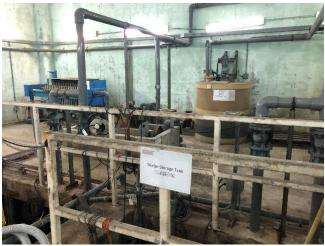
Photo 36: Sludge Storage Tank within the Wastewater Treatment Plant
