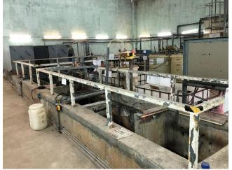
Photo 34: Effluent Well within the Wastewater Treatment Plant
