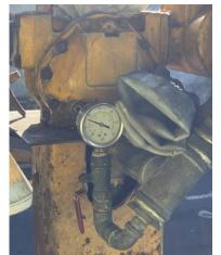
Photo 17: Pressure Meters for Daily Oil Spillage Inspection
