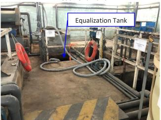
Photo 37: Equalization Tank within the Wastewater Treatment Plant
