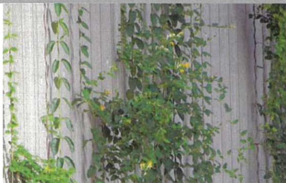
位於政府總部以鋼線作支撐的垂直綠化 Planting with wire support at Central Government Offices
