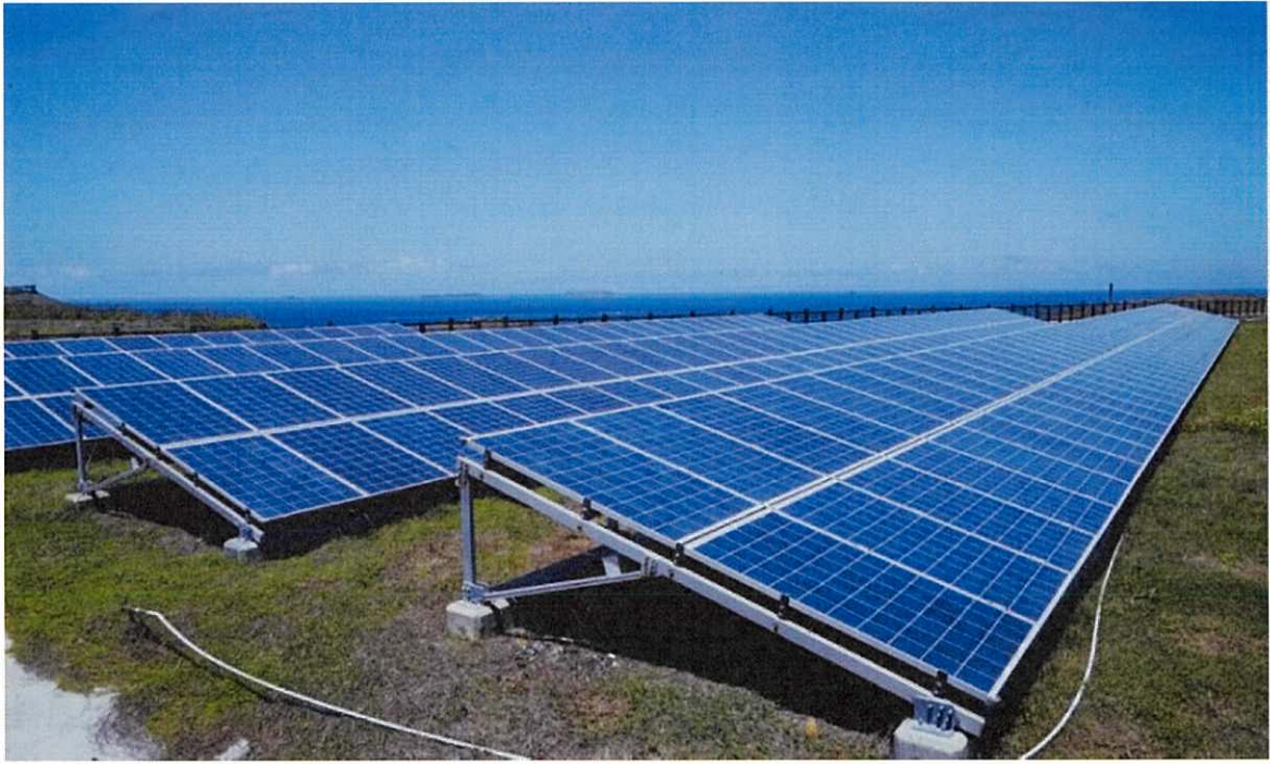
Figure 5, sample picture of solar panel with bracket of 1.5m high and vegetation. (Site B)
