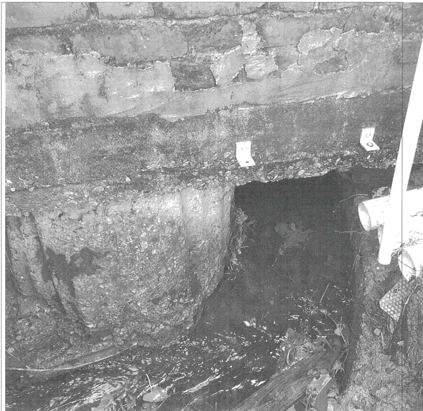
View 1 Existing 900m depth box culvert
