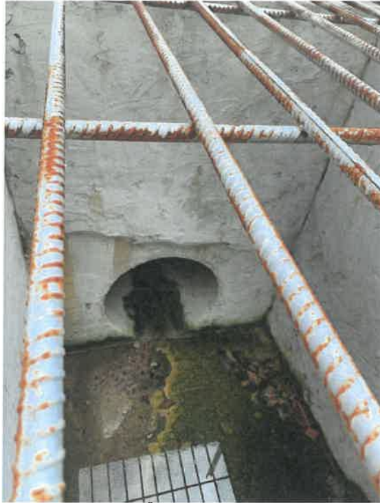
PHOTO NO. 7 Existing 600mm Pipe Inside Existing Catchpit C1 Discharging Water to the Existing Public Inlet Structure
