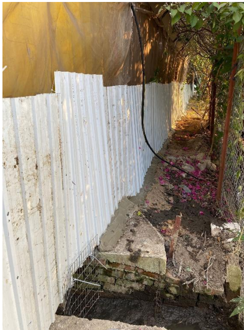
(e) U-channels and spaces between the ground and the structures on the site are sealed off from access by rodents.
