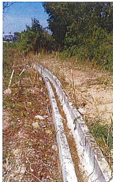
Photos 4&5: Clearance of U-channel and curb maintained
