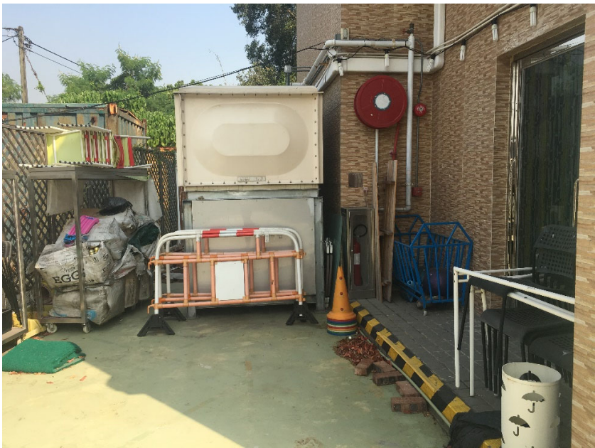
General View of F.S. Tank
