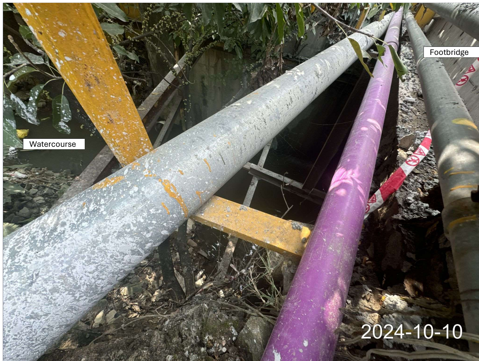
Figure 3-7: Photo of the Existing Watercourse underneath Footbridge
