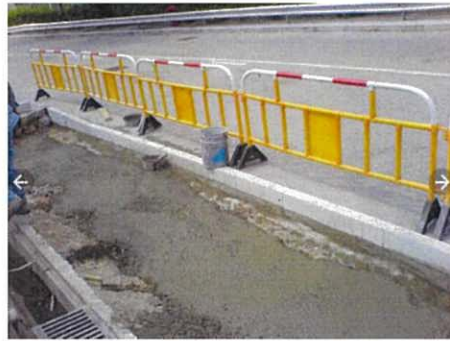
(4) Concrete paving
