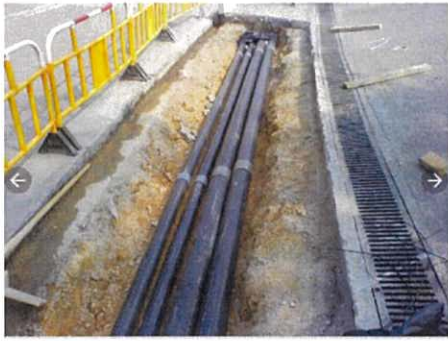
(3) Laying of Spare PVC Duck
