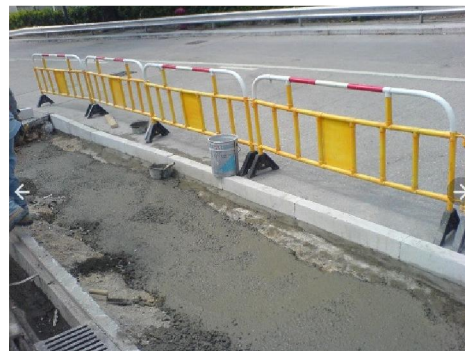
(4) Concrete paving
