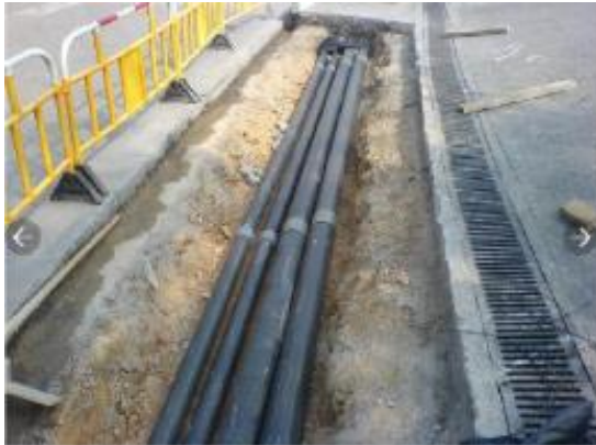
(c) Layout of spare PVC duct
