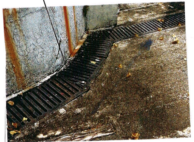
300mm surface channel at residential house front gate
