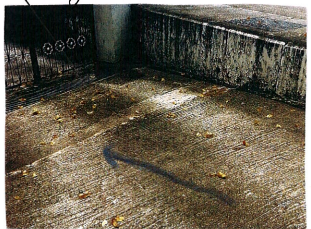
300mm surface channel at residential house front gate
