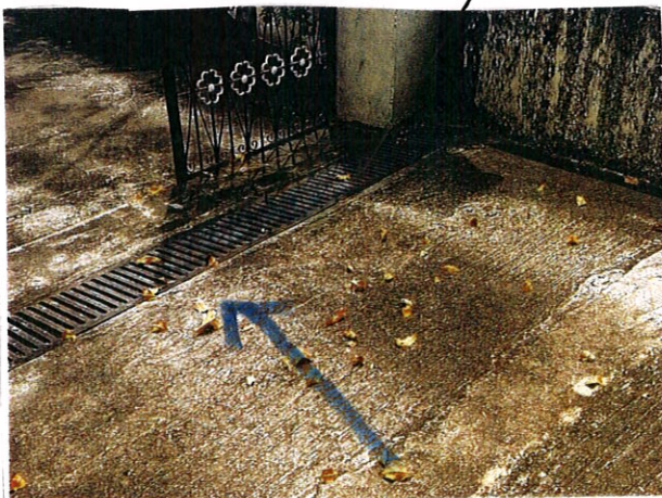
300mm surface channel at residential house front gate
