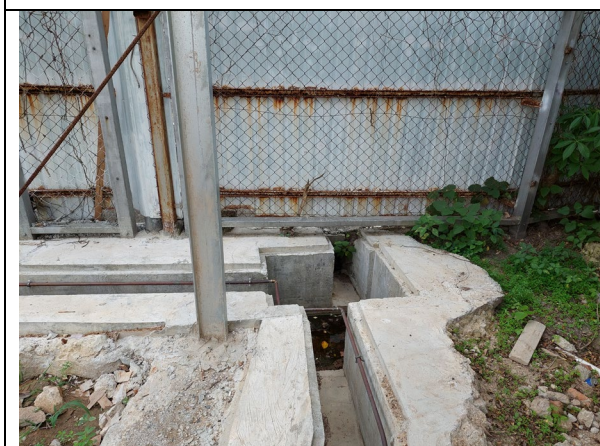
Plate 7 – Existing terminal catchpit with desilting facility at the southwest corner of the subject site
