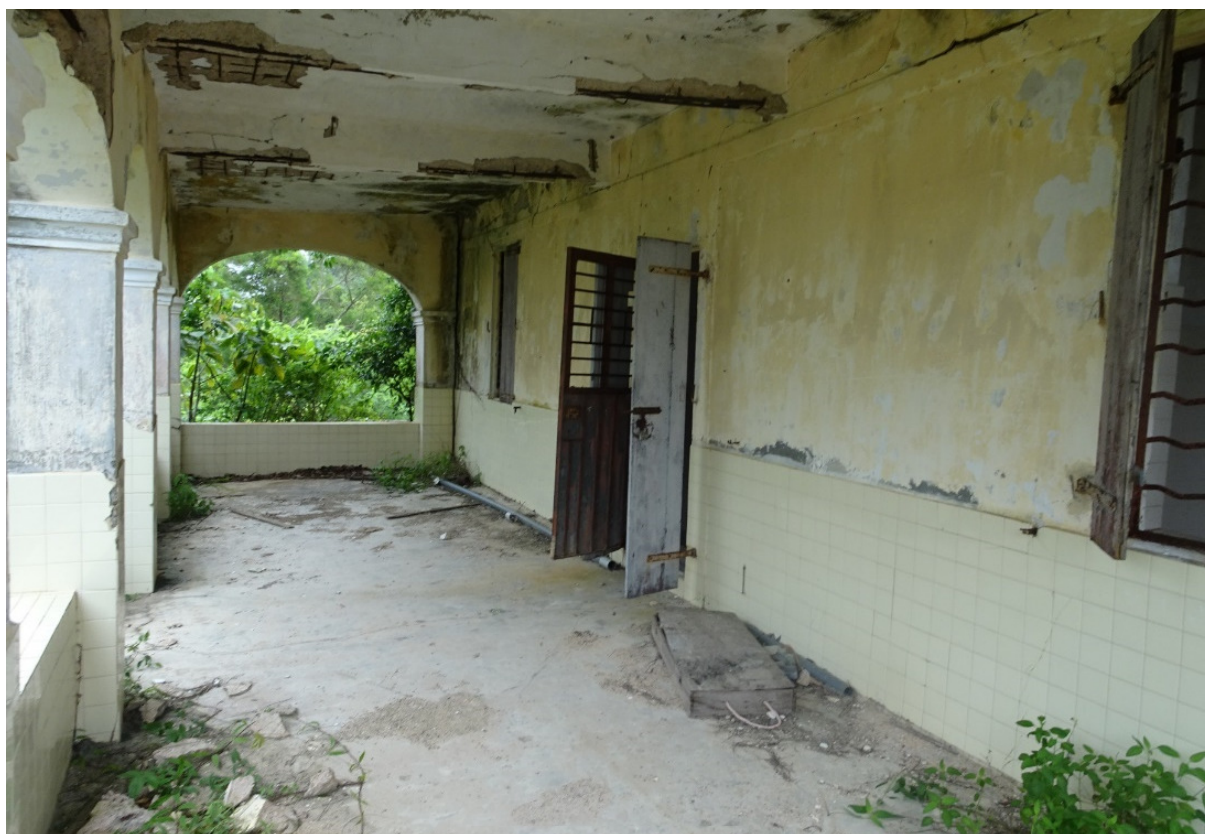
(現有屋宇內部情況) ( Interior condition of existing house )
