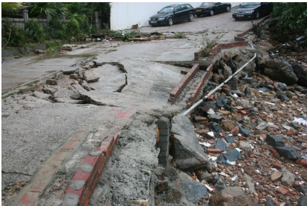
Photo 10: Collapse of Hiu Po Path during the Typhoon Hagupit (Photo taken on 23.4.2008)
