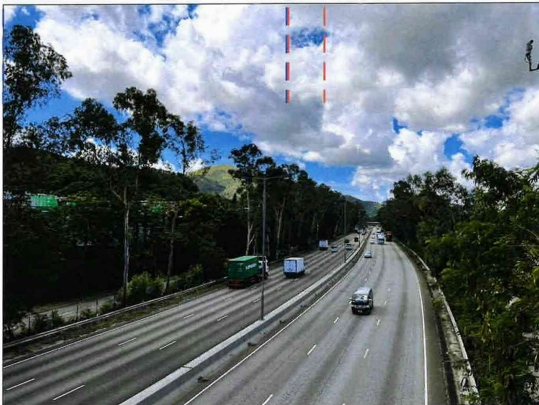
Existing condition (Scheme A)
