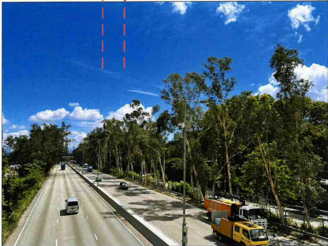
Existing condition (Scheme A)
