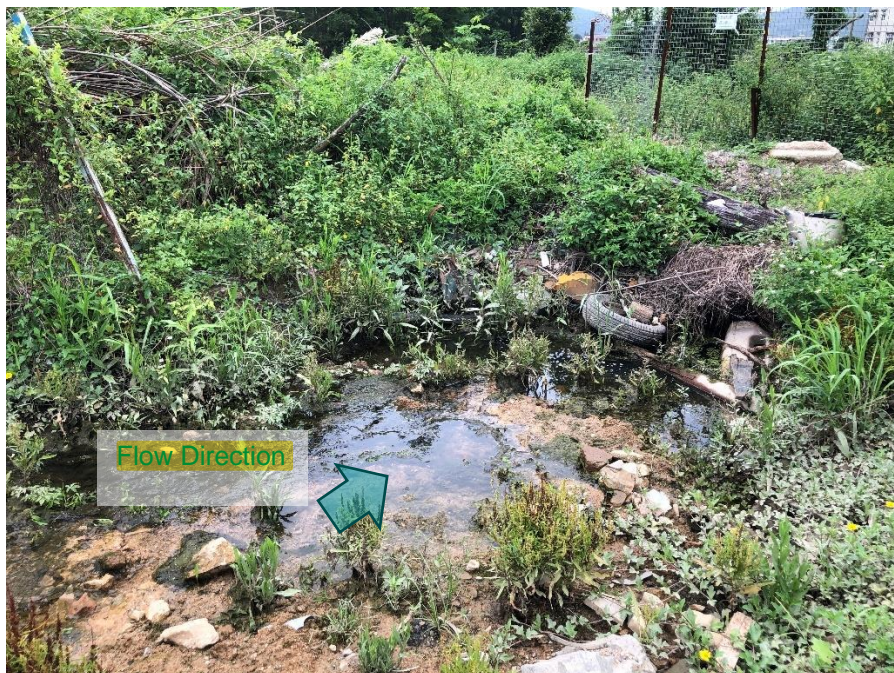
Figure 3.2: Blockage of the Northern Channel Taken on Site
