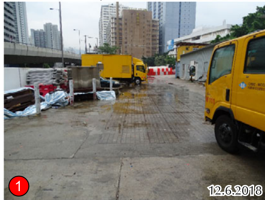
Existing removable drainage covers on ramp down to box culvert
